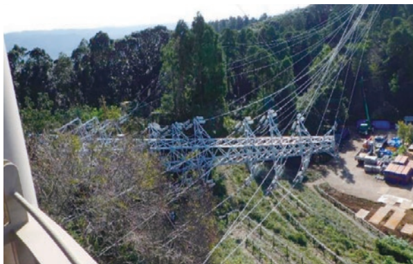
Transmission Tower Collapsed by Typhoon Faxai
