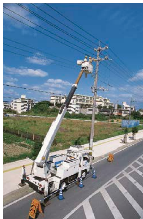
Power distribution equipment (Okinawa Electric Power Co.) Maintenance work in preparation for a typhoon
