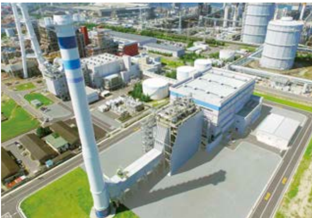
Unit 2 of Sakaide Power Station (Shikoku Electric Power Co.) Reentered service after conversion from oil to LNG-CC in August 2016.
