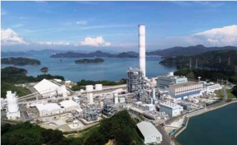
Osaki CoolGen Project Ownership: J-POWER 50%, Chugoku Electric Power Co. 50% Type: Oxygen-blown IGCC Output: 166MW
