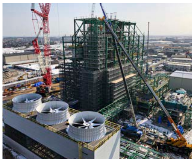
Yonago Biomass Power Station
