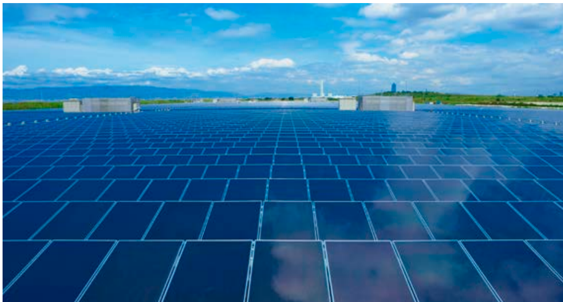
Sakai Solar Power Station (Kansai Electric Power Co.)
