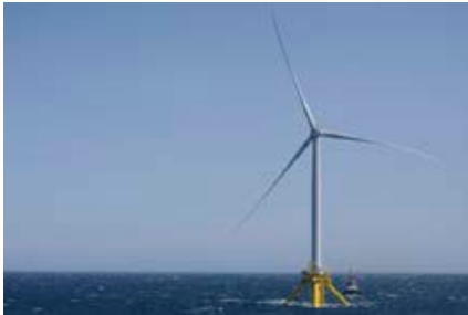
Installed in the Metcenter Test site in Norway
