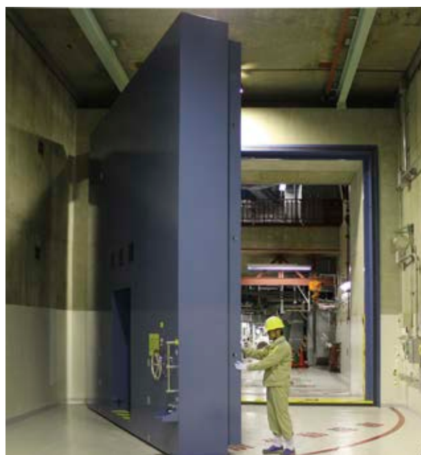
Entrance door and equipment hatch of Tokai II Power Station (The Japan Atomic Power Co.) made watertight Tokai II Power Station entered operation in November 28, 1978
