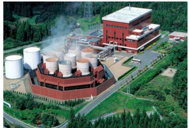
Yanaizunishiyama geothermal power station (Yanaizu-city, Fukushima) (Tohoku Electric Power Co.)
