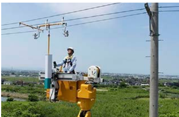
Assist Arms (Hokuriku Electric Power T&D)
