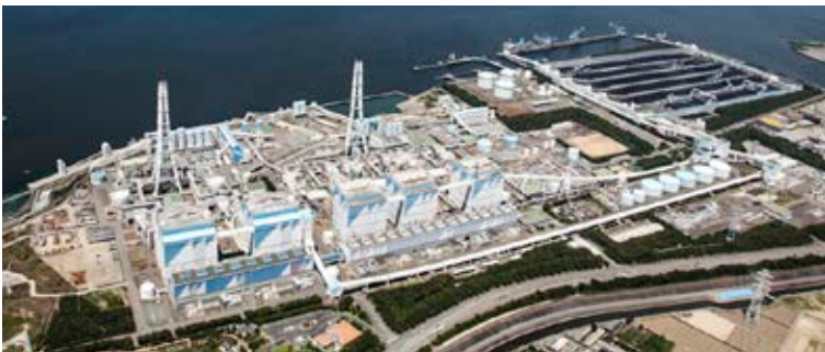
Hekinan Thermal Power Station (JERA)
