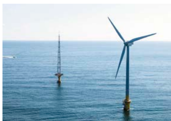
Choshi Offshore Wind Power Station (TEPCO Renewable Power)
