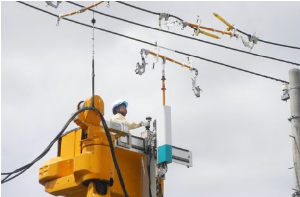
Assist Arms (Hokuriku Electric Power T&D)
