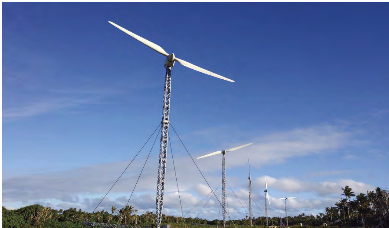
Folding wind turbines being promoted by Okinawa EPco delivered to Tonga (Okinawa Electric Power Co.)
