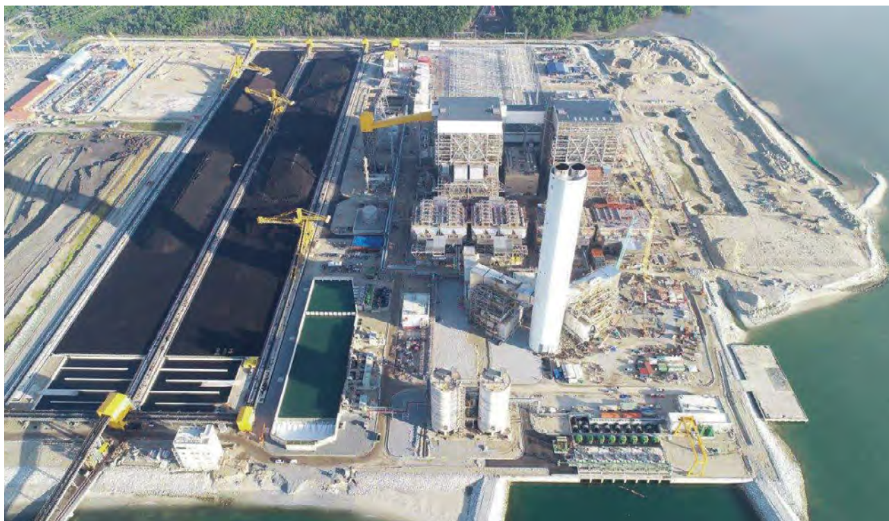
Jimah East Coal-fired Power Plant in Negeri Sembilan, Malaysia (Chugoku Electric Power Co., TNB, and Mitsui & Co.) Jimah East is a USC plant with an output of 2,000 MW (1,000 MW × 2 units). Commercial operation started in 2019.
