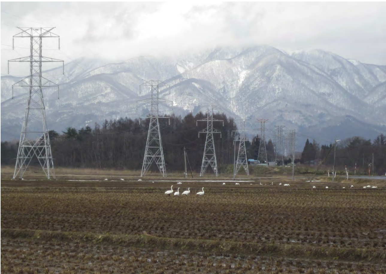
154kV Inawashiro Kyu-kansen transmission line (TEPCO Power Grid) Constructed in 1914 with the third longest (225 km) transmission line in the world at that time. Still in commercial use more than a century later. The transmission towers were manufactured by American Bridge.
