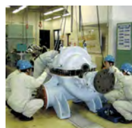
Pump disassembly and inspection
