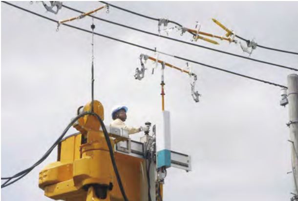
Assist Arms (Hokuriku Electric Power Co.) Hokuriku Electric Power Co. has been working with universities and manufacturers to develop "Assist Arm" robots for use by power distribution workers. In the near future, these will reduce labor requirements and improve efficiency by automating some work.
